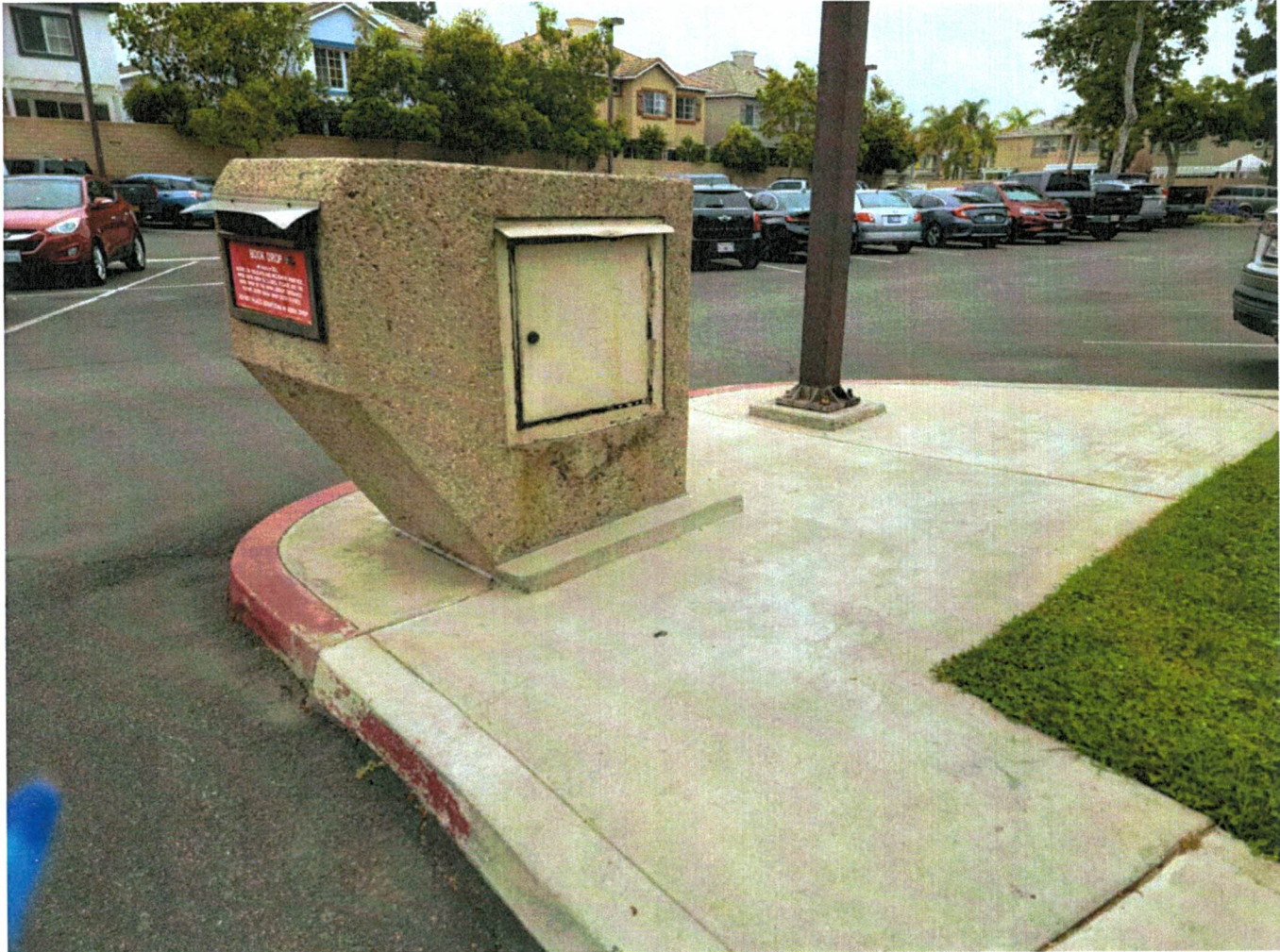
Figure 6 - Photo of Book Drop to be demolished
