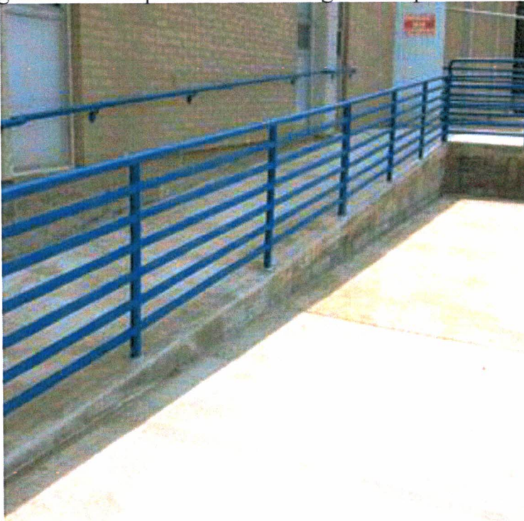
Figure 9 - Example of ADA railing for ramp
