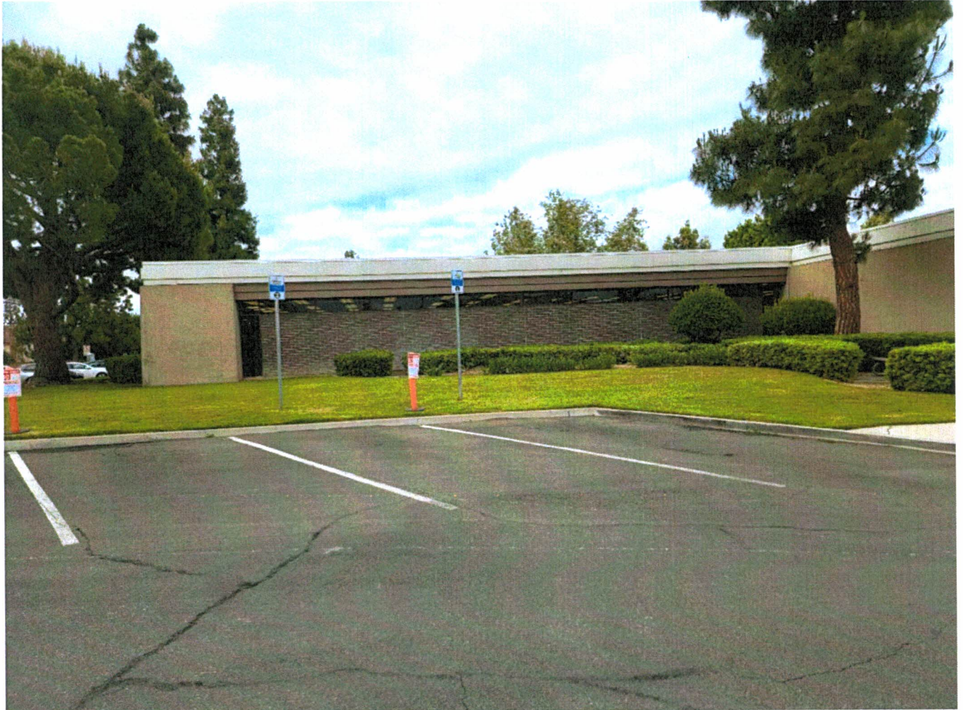
Figure 1 - Photo of northside Placentia Library District Building and parking lot spaces for potential EV Charging Station
