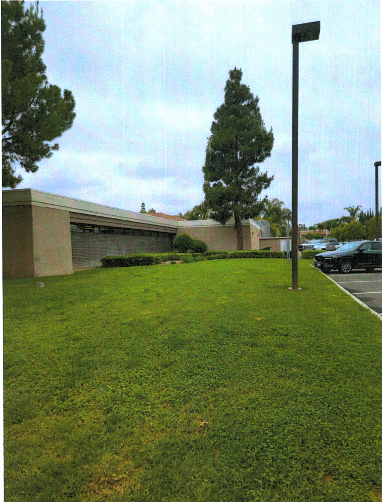
Figure 3 - Photo of northside Placentia Library District building taken from the eastside viewpoint for the new outdoor library facility.
