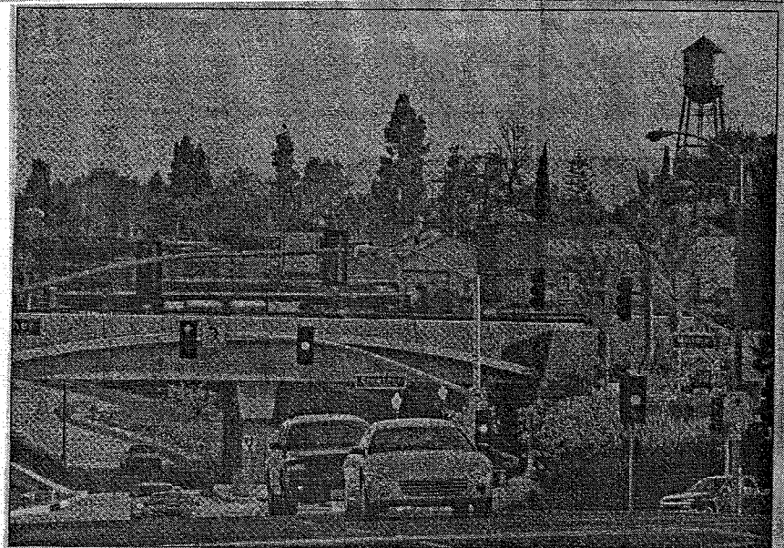
DON KILBURN Los Angeles Times ROLLING ALONG: The Melrose Street underpass, constructed as part of Placentia's ill-fated OnTrac project to rebuild the Burlington Northern, Santa Fe corridor, allows vehicle traffic to flow.
